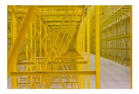
All Structural Steel ASTM A529, Grade 50.
